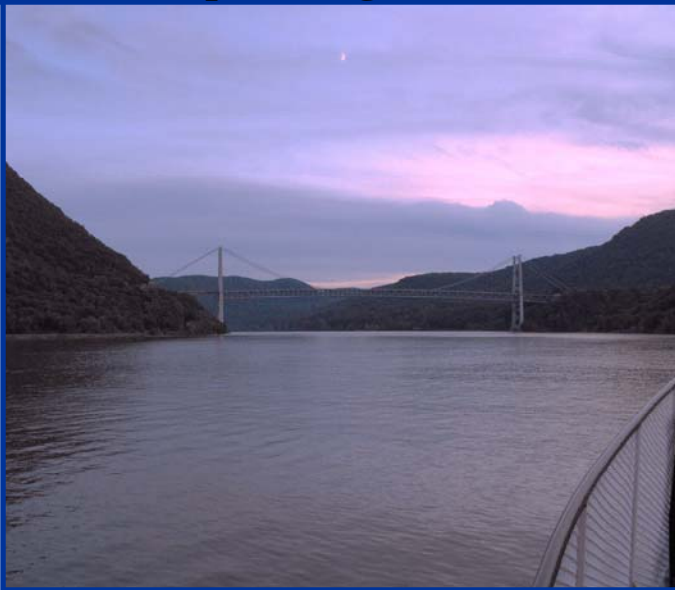
Bear Mountain Bridge over the Hudson River south of West Point
